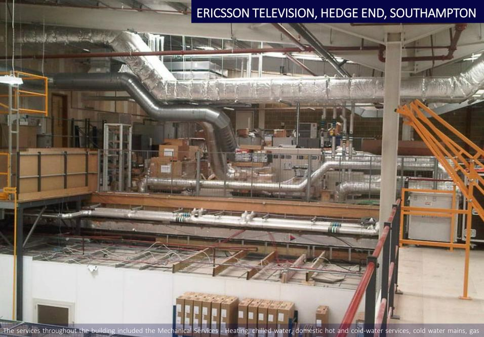
services throughout the building included the Mechanical Services - Heating, chilled water, domestic hot and cold-water services, cold water mains, gas services, VRV air conditioning, close control cooling, supply and extract ventilation, dedicated extract systems, toilet ventilation, leak detection systems and building management controls system. Electrical Services - Small power, mechanical services power, switchroom upgrades, lighting, lighting control and data cabling installation
