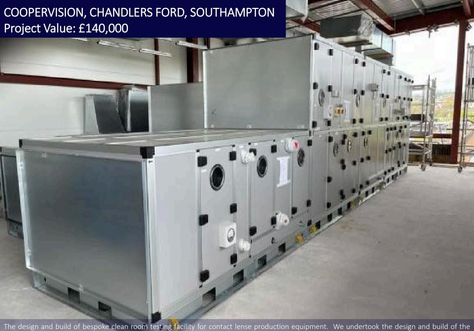
mechanical and associated electrical services including hepa filtration, stringent, pressure and temperature control amounting to certification to Class 100,000. The clean room was constructed within an existing facility providing some 350m2 of clean room space
