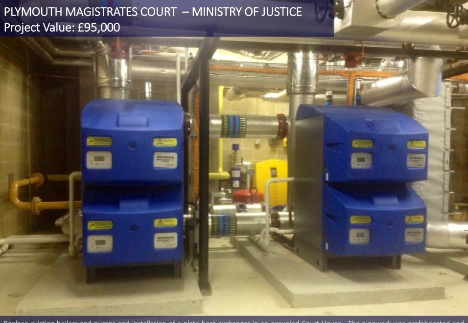
Replace existing boilers and pumps and installation of a plate heat exchanger in an occupied Court House. The pipework was prefabricated and installed during a weekend shutdown, ensuring the system was fully operational on Monday morning. The works also included modification to the flues and control system
